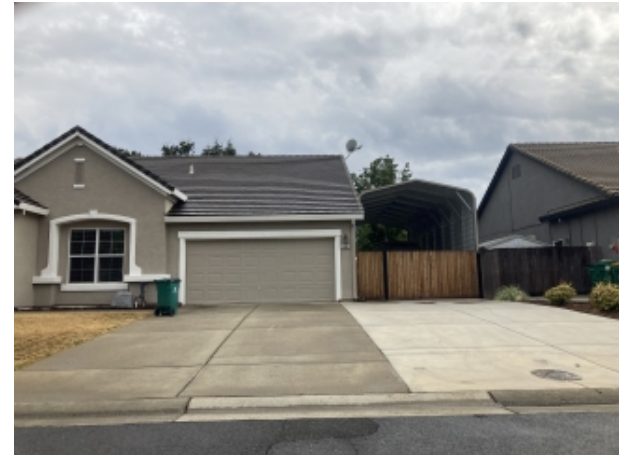
Uploaded on: 09/22/2022 - CC&R Pic Un-approved steel structure on lot
