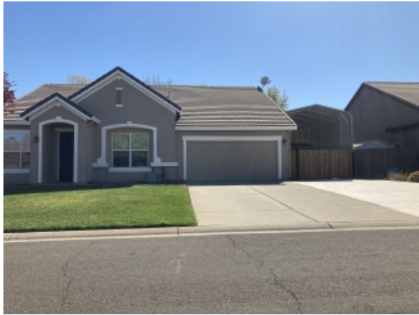
Uploaded on: 03/25/2022 - CC&R Pic Large Aluminum storage structure without approval and within setbacks
